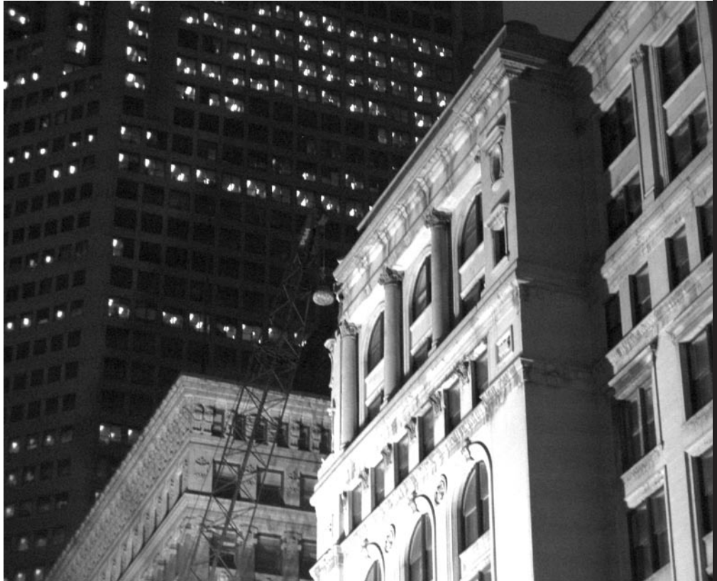
Top: With a wrecking ball poised above its corner, the Century Building waits. Bottom: A local architectural salvage company at work, with permission to remove the historical ornamentation from the Century Building prior to demolition. Both images by Alan Brunettin ©2004.
