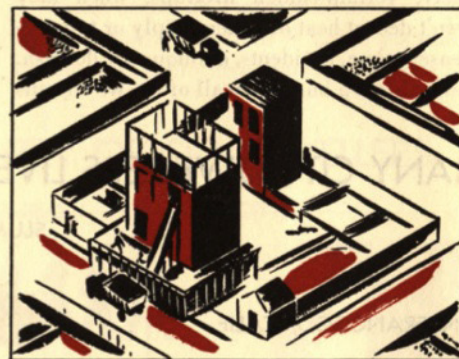
BUILDINGS ARE RAZED
